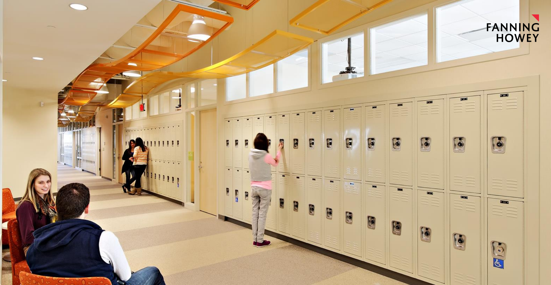
Double tier locker in the corridor with transoms above
